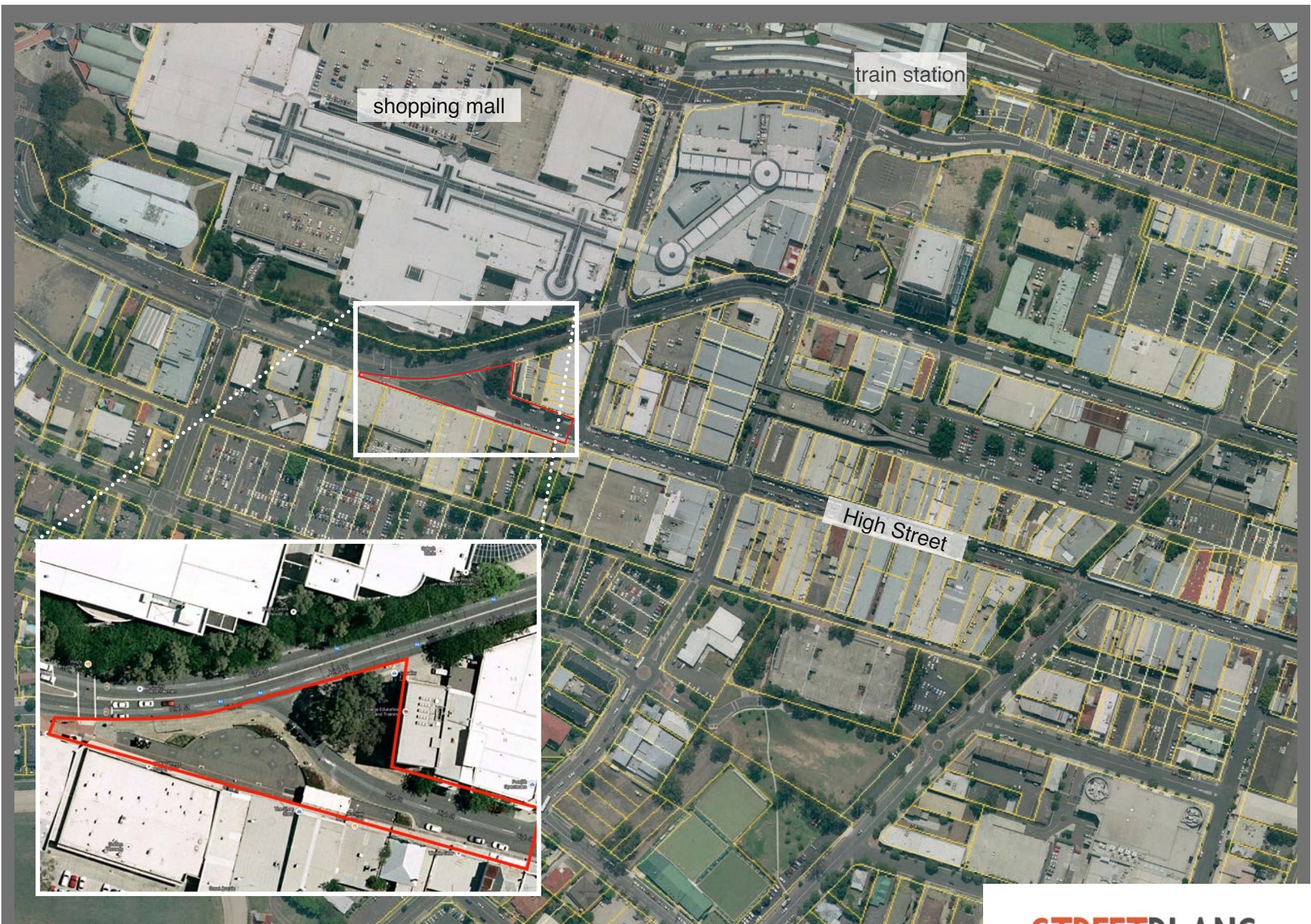
Aerial photo of project site location within the city centre.
